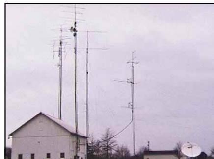
Tom Whitted, WA8WZG, in EN81, uses this impressive collection of antennas—and more—to cover every
