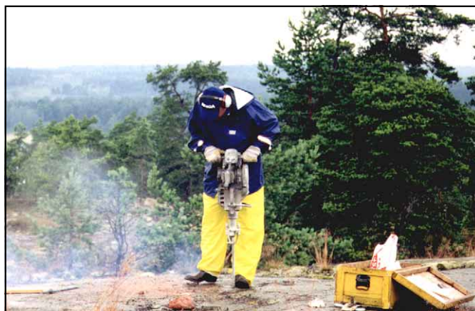
Juha, OH1JT, drilling a hole for a 12-inch bolt.
