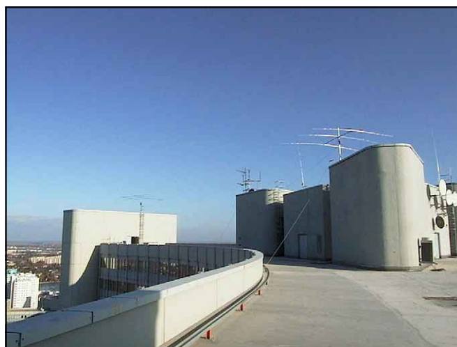
The 4U1VIC antenna farm is located on the roof of the Vienna International Center. The only permanent amateur antenna is an R5 vertical. Any additional antennas must be installed immediately before—and taken down immediately after—each operation.
