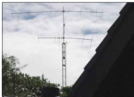
The resort's permanent antenna farm includes an 8-element 6-meter Yagi, a Force 12 C3 and several wire antennas.
