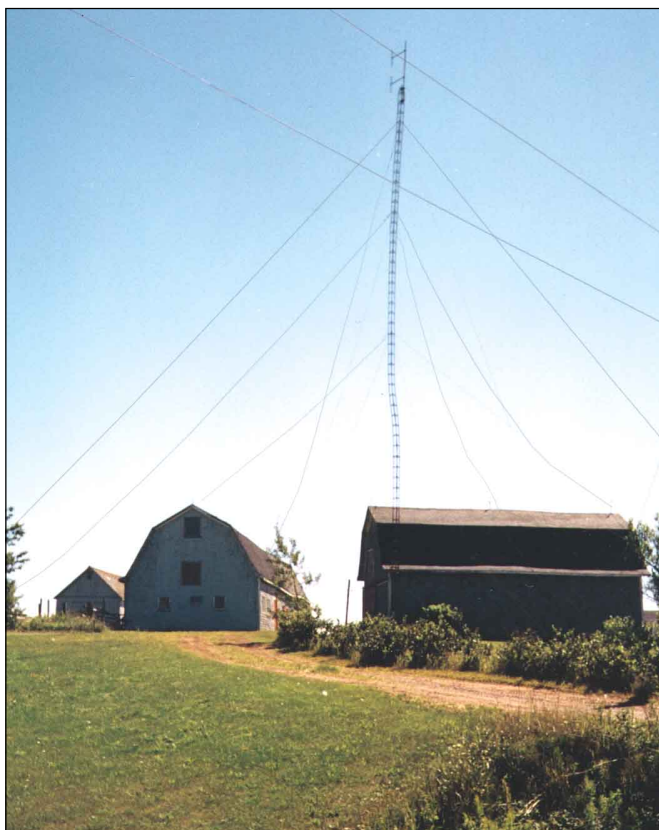
Here's the alternative to careful tower guying! Randy, WA2OMT, spotted this injured installation while vacationing on Prince Edward Island, Canada. No, this isn't an amateur tower, but it's a sight to give any ham food for thought.
