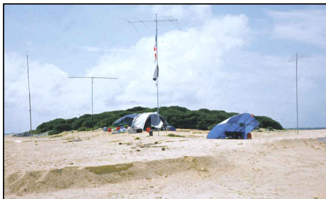
The completed CW/RTTY/WARC band site consisted of a FinnFet tribander, a two-band WARC beam, a 6-meter beam, an elevated R7 vertical and a low-band dipole. The protection of the blue tarp provided effective protection for the Suzuki generators from the nightly rainstorms.
