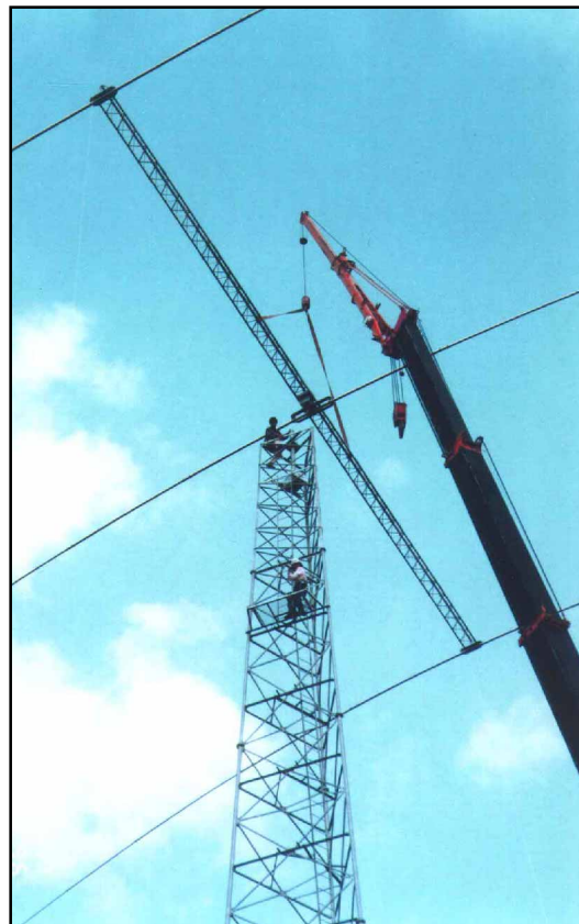
Three elements on 80 meters—believe it or not. Seeing is believing! You're looking at the installation of a full-sized 80-meter Yagi at the station of Kan Inshu, 7J4AAL, in Hiroshima, Japan. Setting the giant antenna in place on its 140-foot tower required a heavy-duty construction crane and a crew of 12.
