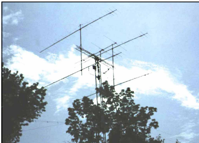
Antennas at W8WN—quad array of KLM 16 LBXs for 144 MHz, 4-element Yagi for 50 MHz, 10-element X-Yagi for 432 MHz—all on the same az-el mount.
