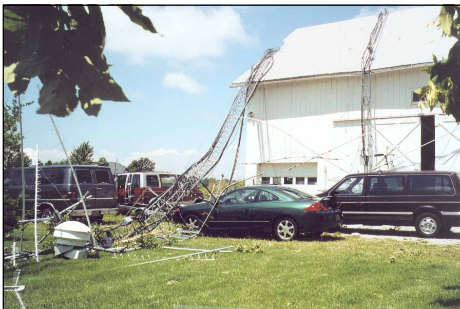
The VHF/UHF/microwave towers of Tom Whitted, WA8WZG, looked like limp spaghetti draped over his barn after a tornado passed near his home on Lake Erie this past July. The tornado traveled about 3 miles, but never got closer than 80 to 100 feet above the ground. Only trees and towers above that height were damaged.
