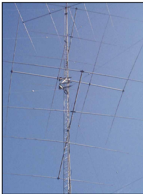
The swinging gate mount and Yagi (middle portion of photo) completely installed on the tower.
