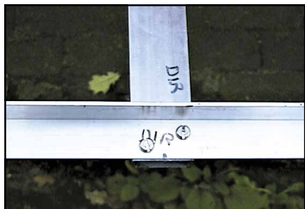
An angle section bolted to the boom.
