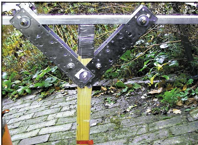
Temporary plates for the boom-to-sub mast.
