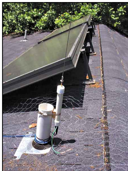
A sheet of chicken-wire screening can be laid beneath the antenna and connected to the antenna ground to stabilize the fields around the antenna to further reduce noise coupling. Chicken-wire screening in rooftop installations is generally hard to see from the ground.
