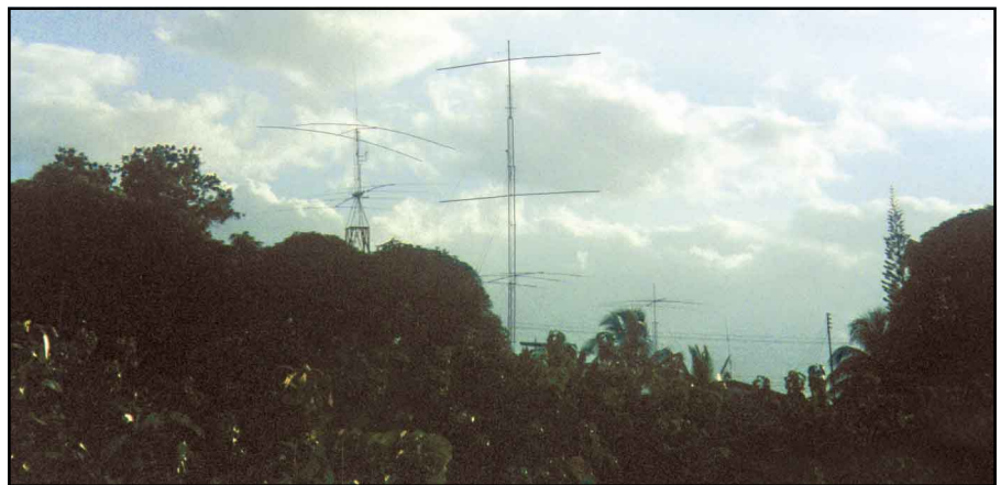
The Hillview Gardens antenna farm. From left to right: a two-element 40 over a four-element 20; stacked six-element, 6-meter beams over a tribander fixed on the States. In the background is a C-3 tribander at 50 feet.
