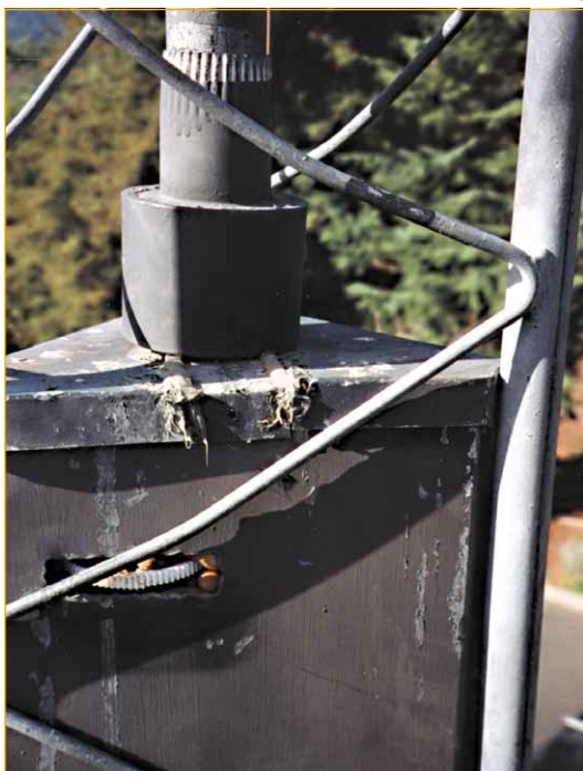
The acorns are visible through the indicator gear opening. The jays forgot one thing: The acorns are easier to get in than to get out!
