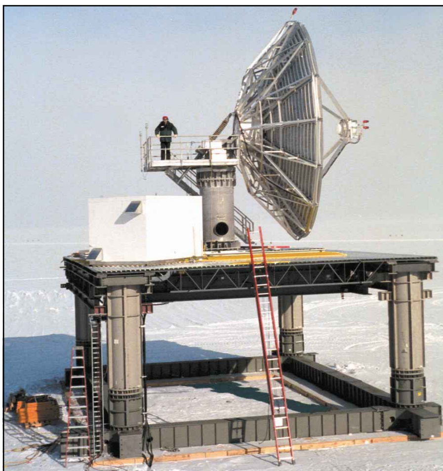
Figure 5—The completed 9-meter reflector, antenna shelter housing RF components and platform comprised over 100,000 lbs of steel before snow backfilling to add additional stabilization. The platform is designed so that a radome can be added at a later date if necessary.
