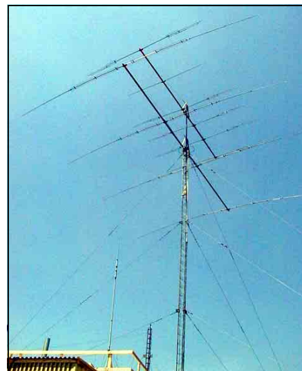
A view of the tallest tower at W6UE. The tower itself is a 50-footer, and it's located on top of a 50-foot building. It supports a 4-element KLM 40 and a KT34XA.
