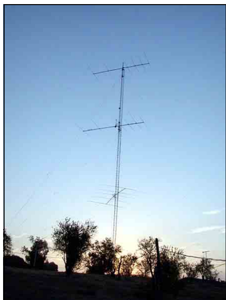
The 15-meter 6 over 6 stack at N6RO.
