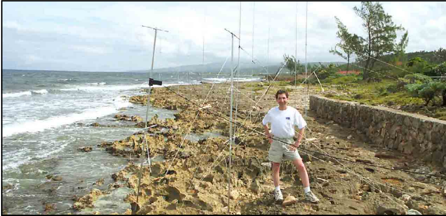
Kenny, K2KW, stands next to a 6-meter Sigma-6 array. A 4-element 10-meter European array, 4-element 15-meter European array, 2-element 80-meter array, and a 160-meter inverted-L are visible in the background.
