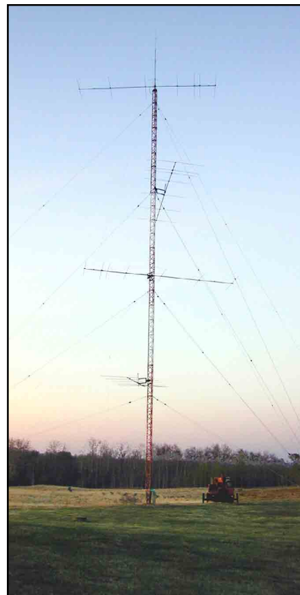
The four-Yagi stack for 10 meters ensures that VE6JY is heard when the band is open.
