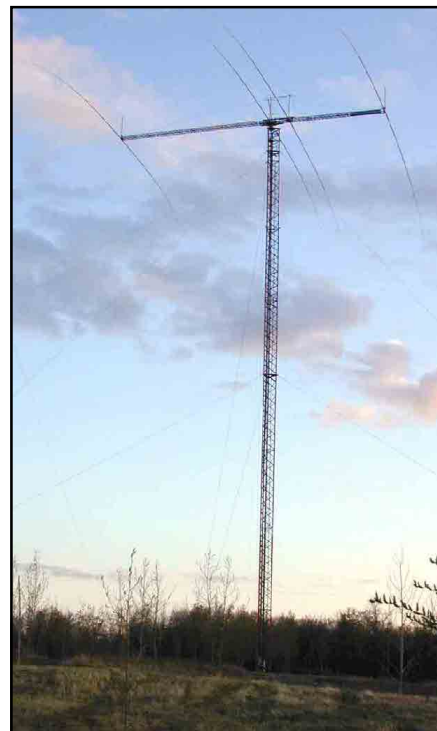
No gin poles for this one: the 80-meter Yagi inspired VE6JY to get a second crane.
