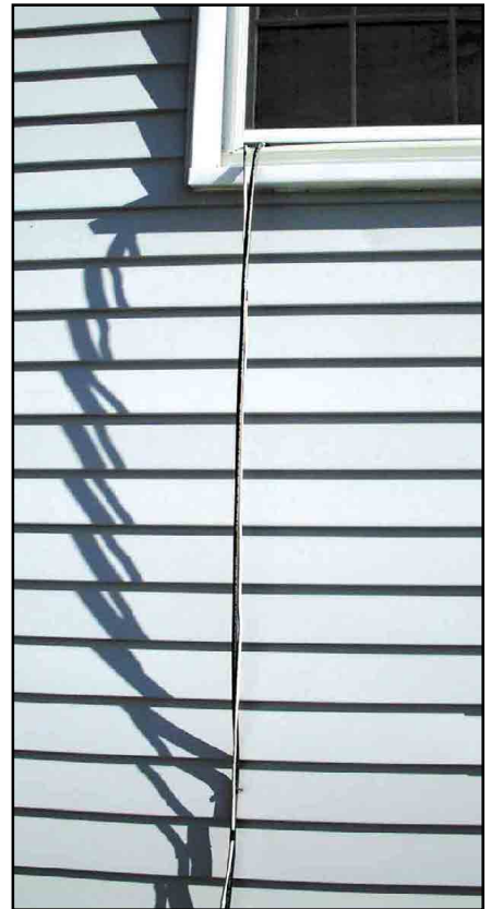
The direct-bury coax makes a discreet jaunt into the bedroom window.
