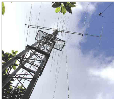
The tower and beams at T88ZZ.
