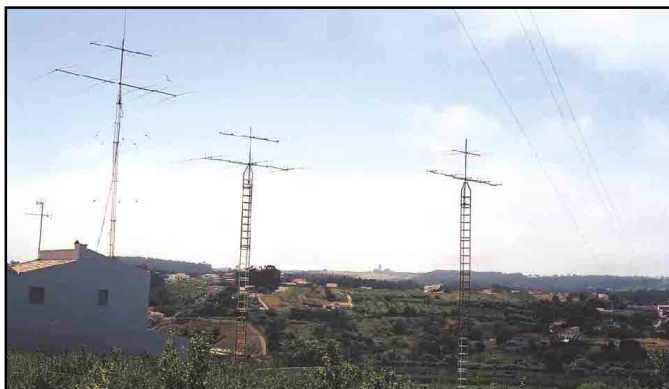
Francisco O. Felizardo, CT1ALF, of Caidas Da Rainha, Portugal, sports an impressive antenna farm: Titanex V160 vertical for 40-80-160, and Yagis for 6 (PKW), 12/18 (Hy-Gain), 15 (PKW), 40 (PKW), 20 (Force 12) and 10 (Force 12) meters.
