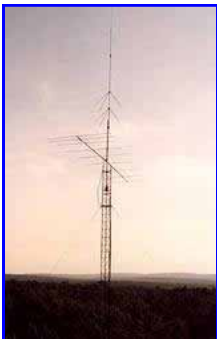
The 49.5', nine element 6 Meter Beam and FM Vertical on their 80' tower
