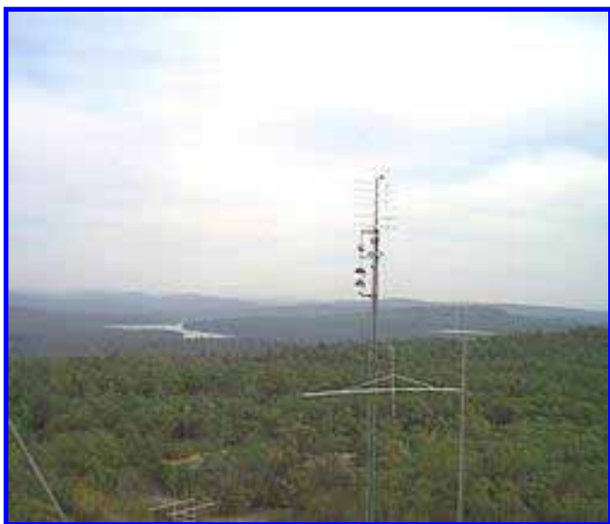
Microwave Tower, 903 thru 24 GHz as seen from the 144 MHz tower. The top antenna is 135 ft above ground.
