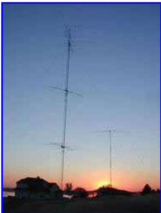
The business end of K7IR - a three-stack of C31XR's at 40/80/120' with a 40-2CD and rotary dipole for 80 on top. Also a plastic owl named Frogman - don't ask. To the right, a small crankup holds a 3-element SteppIR and an 80-meter inverted vee. The big tower will hold all SteppIRs by the end of the year.
