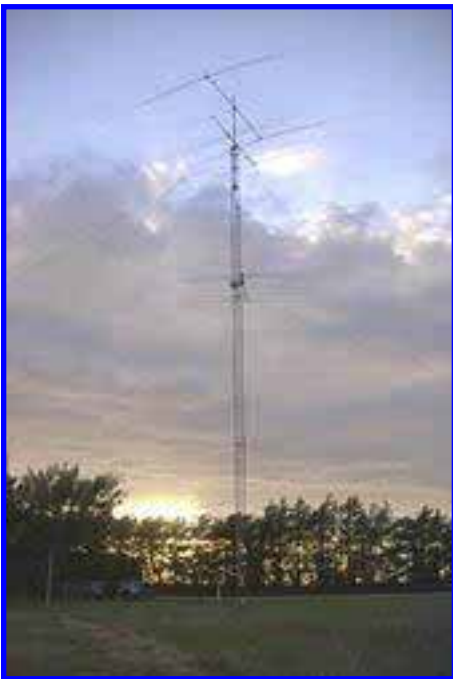
The main tower with stacked yagis and 40. Photo taken from near the 160 tower, used as a halfwave on 80 for this contest.
