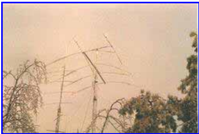
432 stack, KT34A & 2M FM heavily iced
