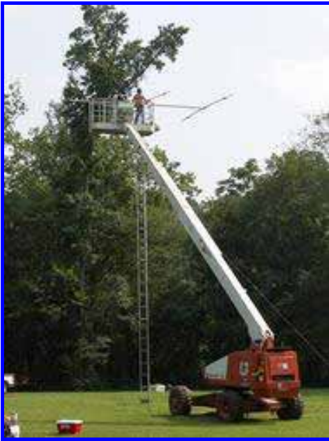
K4TS setup lifting and installing the 10 / 15 Meter Beam using our soon to be UHF/VHF tower. This is the easy way.
