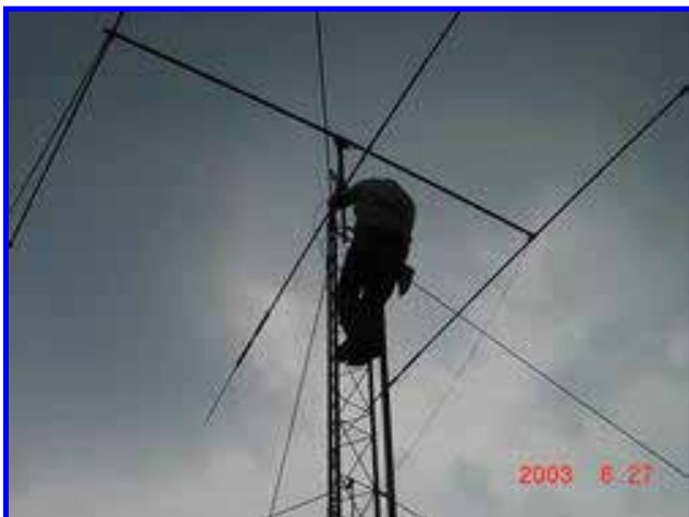
Assembling the A3S tribander.
