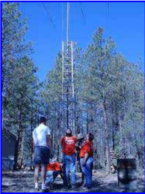
Here we are trying to reach the UHF barrel connector at 15 off the ground to change out a bad feedline. Sure wish we had tested the cable before raising the beam!
