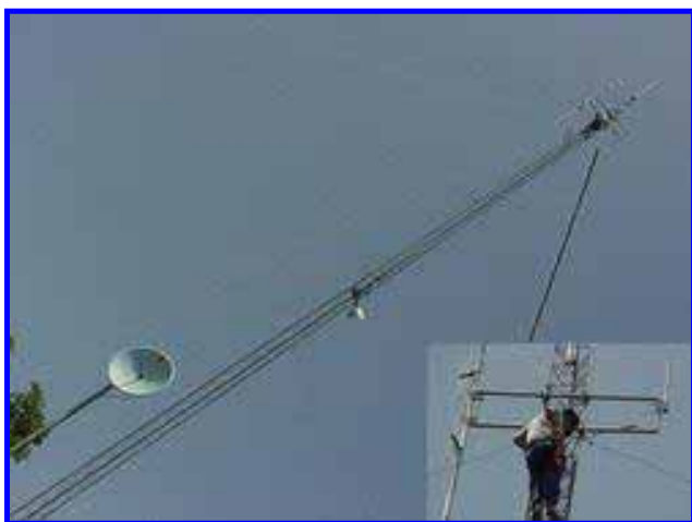
NP4A 200 ft. up installing his 40/80 Delta Loop
