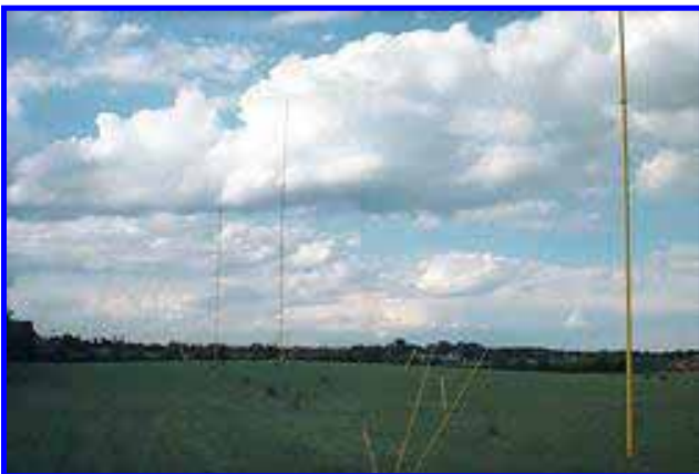
Three 46' towers made of 1/4" wall fiberglass tubing were used as supports for a pair of dipoles. The wire could be swapped to change bands in just a couple of minutes.
