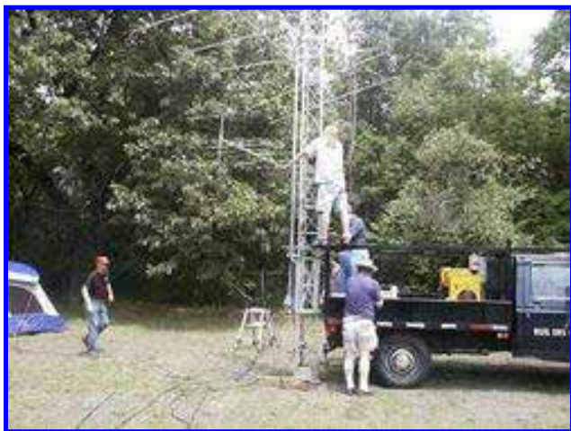
John, N1LEZ, Chris WA1VXH, Dan, W1DMM, and myself, N1KGY, setting up the tower and VHF beams
