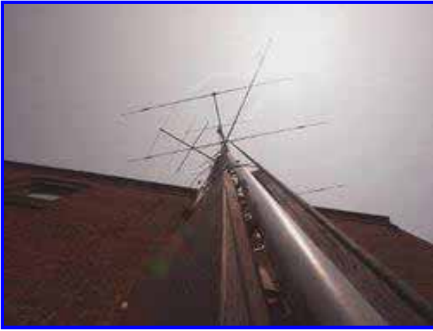
The EOC tribander used by the HF/CW station atop one of the permanent towers, as well as other regular antennas including a G5RV, 6 meter beam, and 2 meter (packet) antennas.
