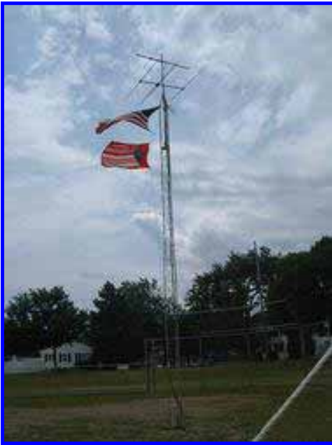
VHF Tower with 2 & 6 meter beams
