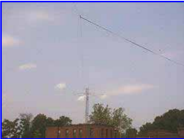
The double extended zepp for 75 meters. This is a new antenna for MARC, and was a big challenge to get in the air at the EOC. At 320 feet long, we needed a shoe-horn to fit it into the available space!
