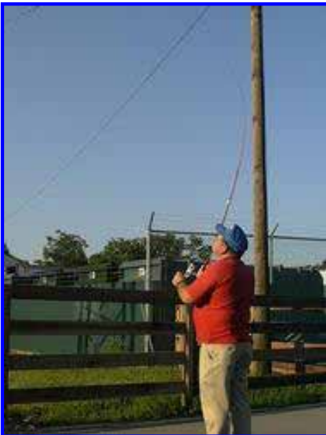
Nope, he ain't fishin. Buddy (KB4EBP) is casting a lead weight over the top of an antenna support. And he is really good at it. Never needed more than one attempt.
