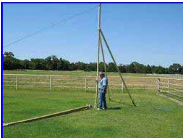
A small boat winch is used on the homemade gin pole.
