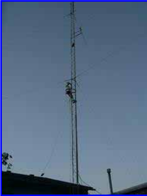
Here is Tandy, KO4OT stringing up the support rope for the 40m vertical. On top of the tower, just out of sight here, was our 2-element beam for 160. Naaaah, just kidding.
