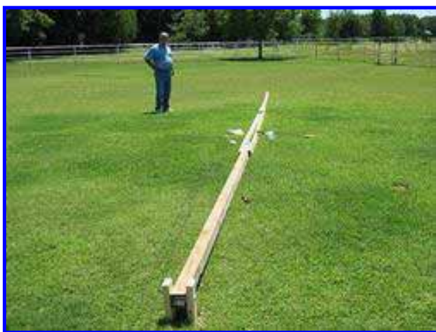
Ready to erect one 44 foot mast.
