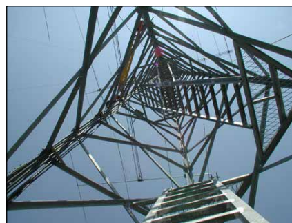
YT6A monster tower. You can also see the tower sections used as the horizontal support for the horizontally stacked 5-element Yagis.
