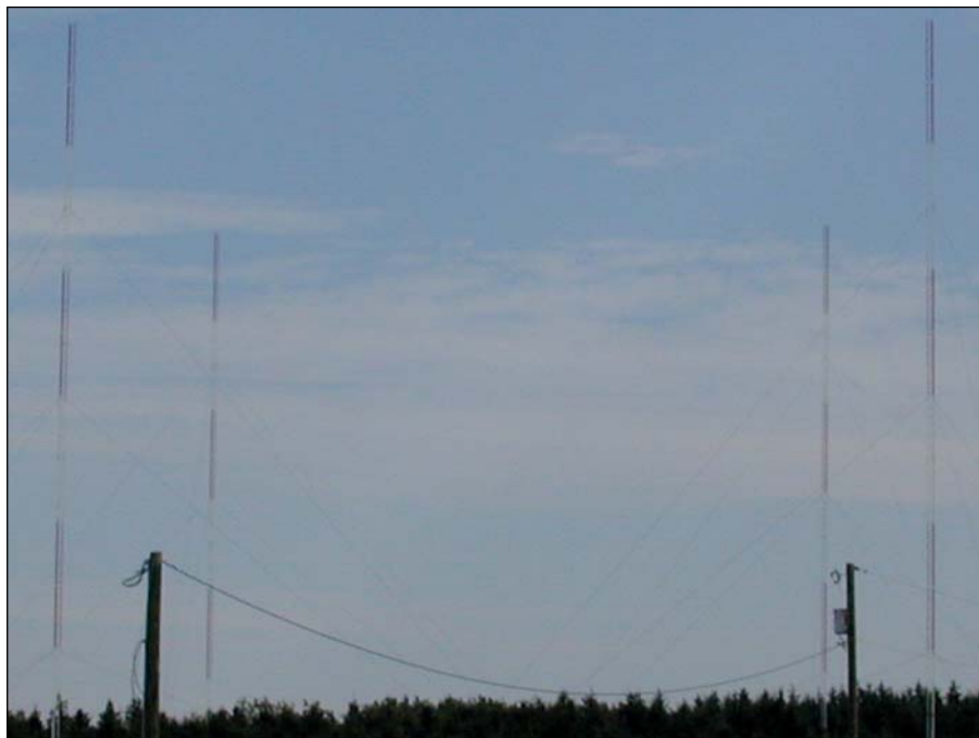
A view of the 4-element VY2ZM 160-meter phased array, showing its rectangular footprint. The radiators are full-sized Rohn tower, on insulated bases, using phillystran guys.
