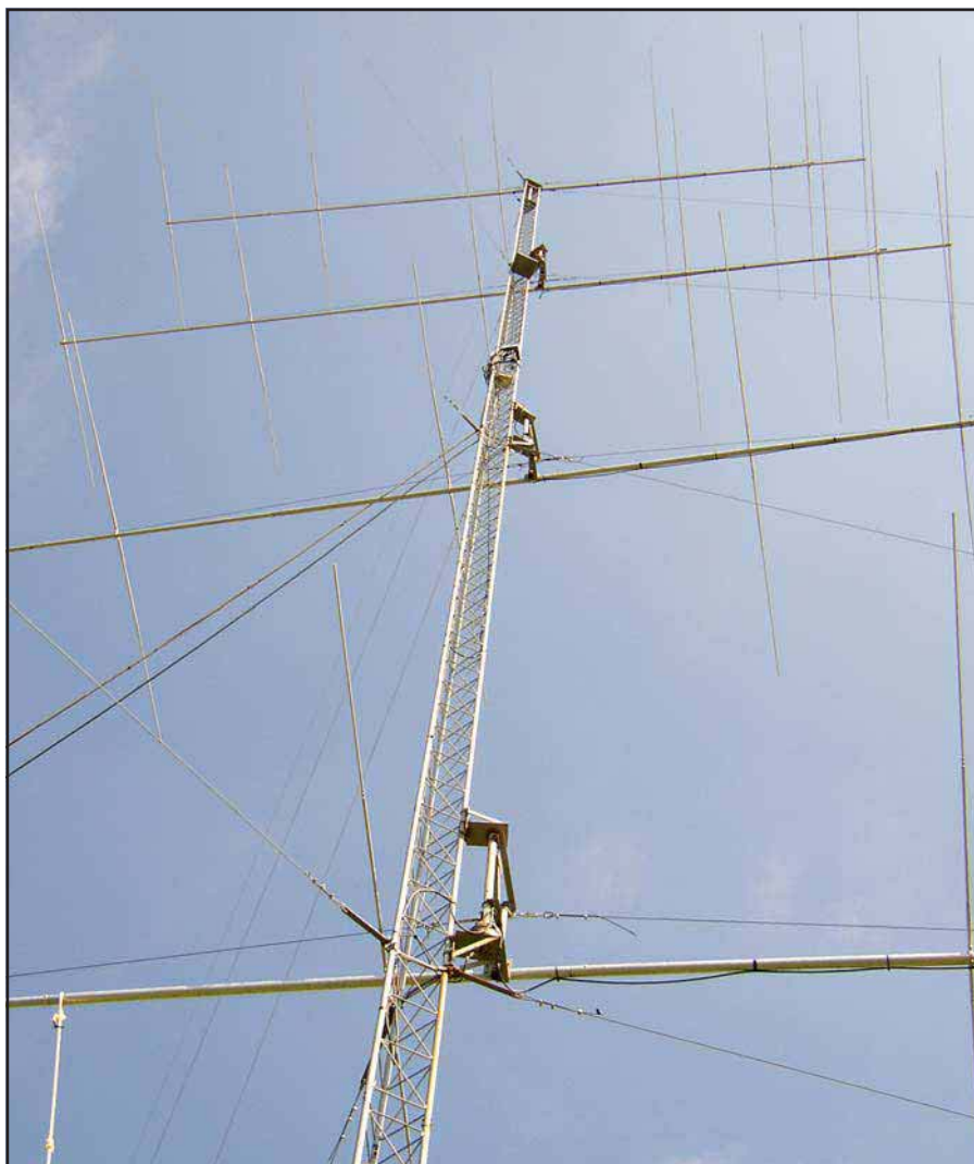
A close-up view of the Yagis and their side-swing arms.
