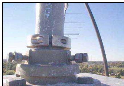
The collar and thrust bearing on the top of the tower.
