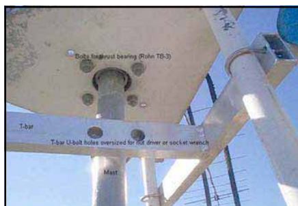
The T-bar just below the thrust bearing.
