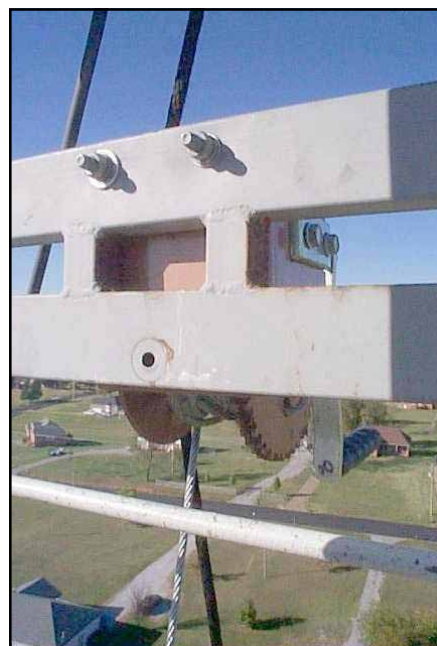
The winch and the frame to which it's mounted.
