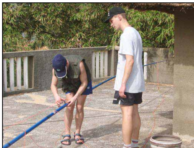
Assembling the 2-element array for 40 meters.
