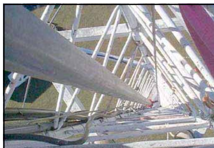
A view down the inside of the tower showing the mast, the pulley at the bottom of the mast, and the cable.
