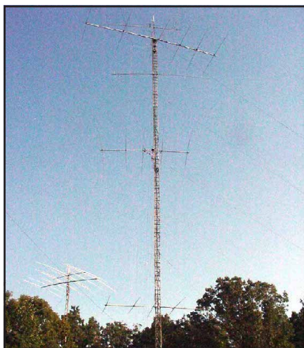
This view shows the 15 meter stack (tower on the right), and the TH7 (tower on the left) with an A3WS with a 30 meter kit above it.
