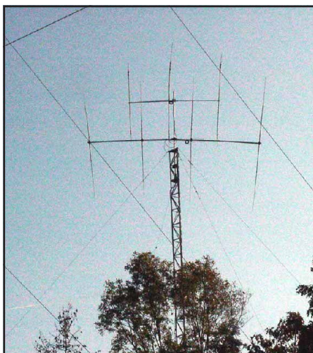
Here is an A3WS with a 30 meter kit at 130ft and a 4 element 20 meter Yagi at 120ft.
