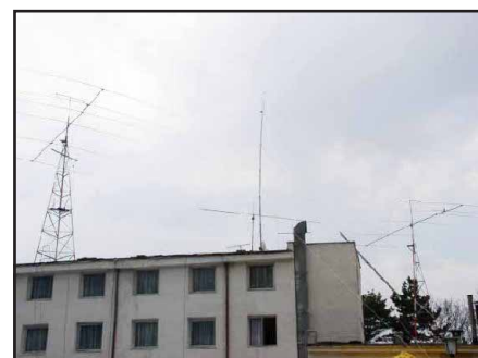
Twenty-meter antenna (left), 80-meter antenna (middle), and 15-meter antenna (right).
