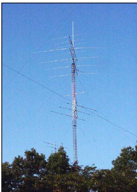
This is the tower behind the old shack. This was the first tower put up at W4MYA in the spring of 1990. It went from 80ft to 100ft in 1992.
