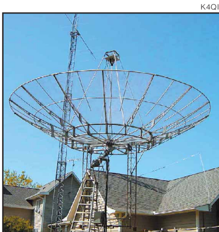
Figure 3—The K4QI 7.5-meter homebrew dish on a polar mount.
