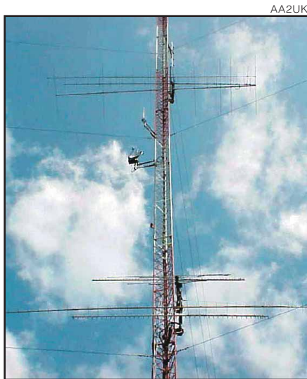
Figure 5—The top of the 95-meter tower at AA2UK with the stacked arrays described in the text.
