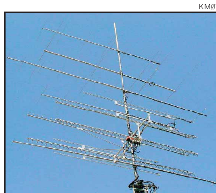
Figure 7—Stacked arrays at KM0T described in the text on a 17-meter crank-up tower.
