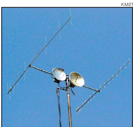
Figure 8—Microwave antennas and FM Yagis on a 13-meter crank-up mast at KM0T.
