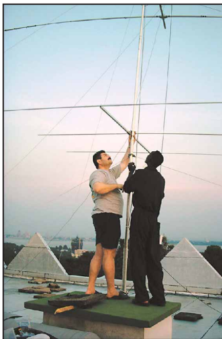
Figure 3—Josep and a Congolese assembling the 6 meter beam.
