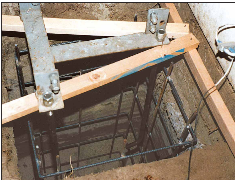
Figure 2—Everything is ready for the concrete pour. Note the tower base-mount J-bolts secured in the base mount for proper alignment.
