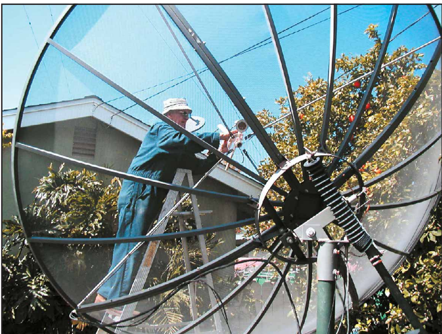
Figure 10—The author adjusting the offset feed support of the modified TVRO dish.
