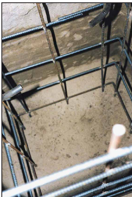
Figure 1—The rebar cage is centered in the excavation. Each leg rests on a 3 inch high preformed concrete pier (not visible).
