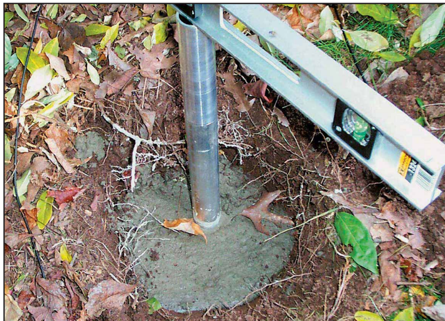
Figure 1—The aluminum mounting tube is anchored in concrete.
