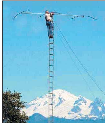
When you get past the magnificent view of the club's namesake, that's Doyle, KC7GX, mounting the 20 meter Yagi for the K7ZC Mount Baker ARC (WA) CW station.
