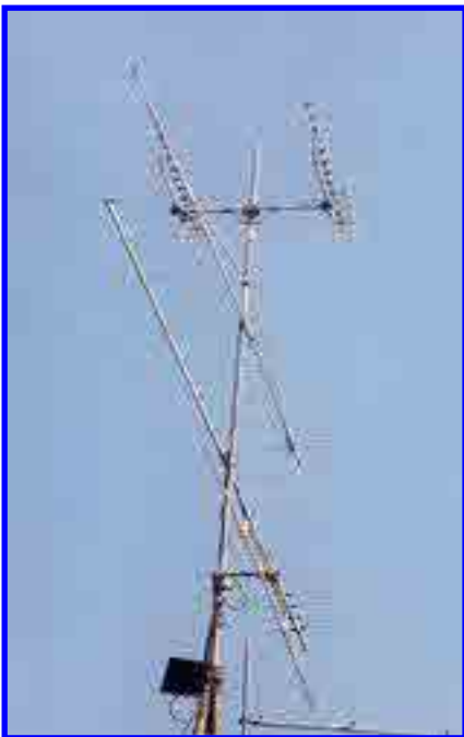
Windmill tower with 144, 222, 432, 1296 antennas.
