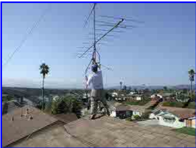
W9EC assisting with 6M yagi installation.
