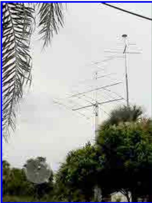
Tower: Mosley Pro67-C3, M2 6M7, M2 222-7WL, M2 440-21ATV, M2 2M12; Rotatable Mast: 1296 45EI Loop, 2304 45EI Loop, 903 18EI Loop
