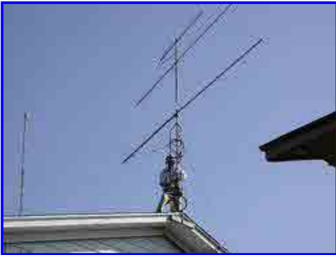
W9EC assisting with 6M yagi installation
