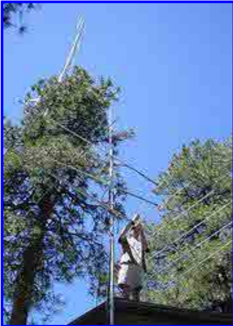
K7MWD wrestling with the six meter beam...
