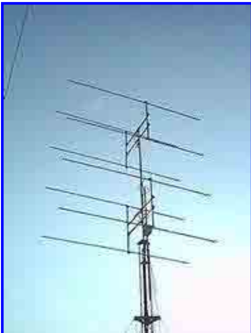
The just completed 8 X 25 element yagis at 106 ft. The tower and antennas were all new this summer.
