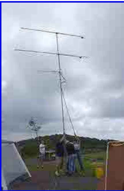
Installing the 432, 2m, and 222 antennas on the rotating mast.
