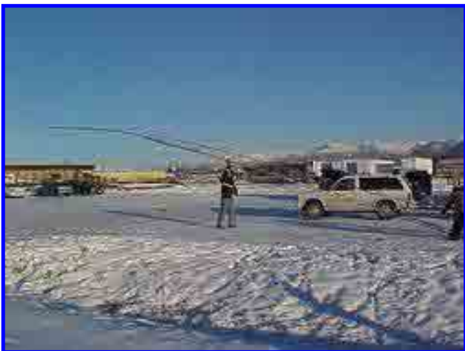
KL7CY "walks-up" the quarter-wave 80m vertical while the ground crew stands by on the guy ropes. The temperature this morning was -5 deg F.
