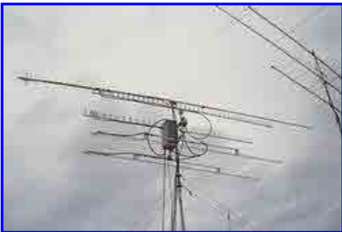
432-3456 stack close up (M2 9WL on top)
