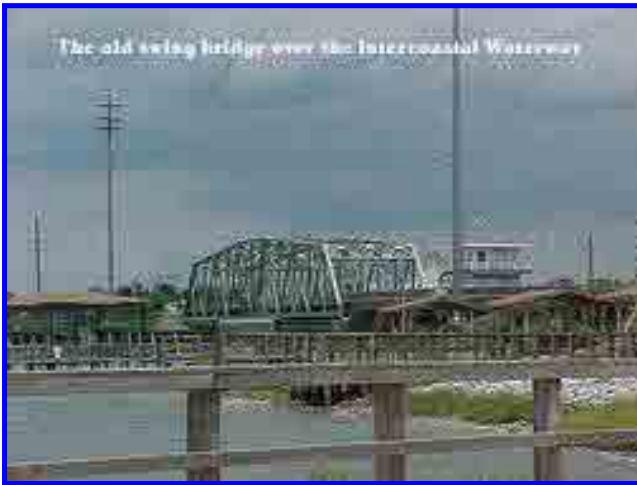
The old swing bridge over the inter coastal waterway on Highway 50 in Surf City, NC
