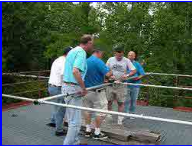
Installing a tri-bander on the smoke house
