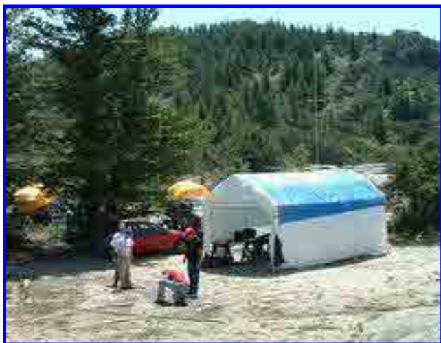
The shelter is up and the beam building crew is busy.
