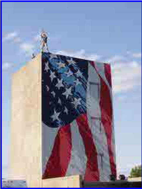
Chad and John hanging antennas
