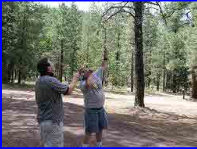
NA7D and WM7A use the classic slingshot method to install a dipole antenna in the tall pines.
