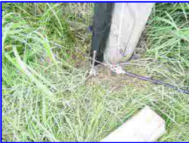
The 40M vertical ground connections. 8 full sized radials connected together with a spare clamp. The pole was placed over a plastic pipe and bound to an old fence post with a plastic tie. Total improvisation on the spot....I love that about Field Day!
