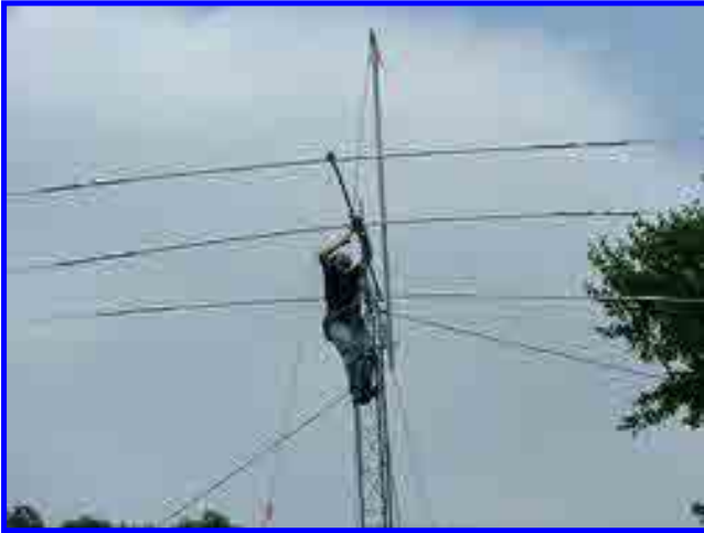
The A3S going up on the tower. Yeah, that's W5UGD up there. Note the sky. (Don't do this at home kids. Rain/Lightning and metal structures do not mix! SAFETY FIRST)
