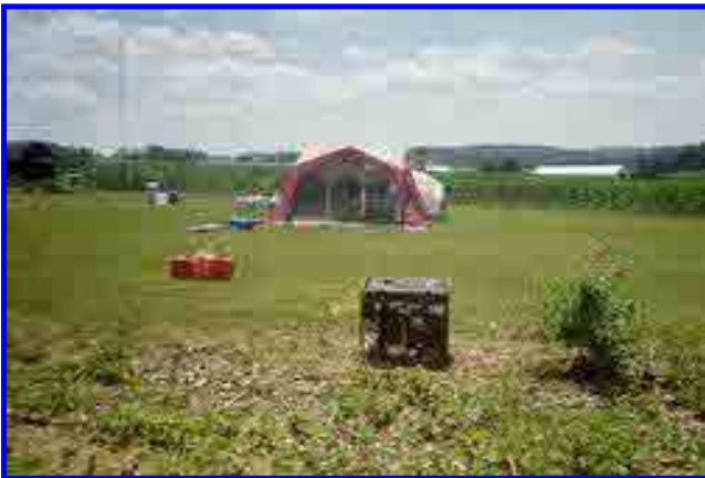
Soggy generator. Works great!!
