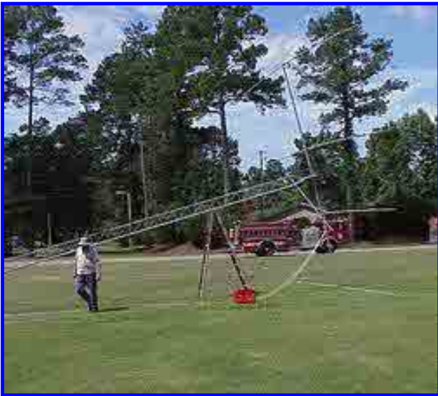
Hoisting the tower with the Tri-Band beam into place.
