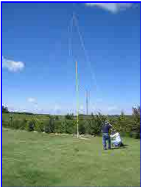
Here's Vlad-N0STL (scratching his head) and Tod-K0TO adjusting the tension on the guys of the North Tower.
