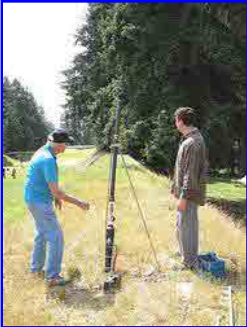
Hal, W7EC, and his assistant- Soren (a new ham without a callsign just yet) aims the Potato Howitzer to shoot a line over the 100 feet high fir trees.
