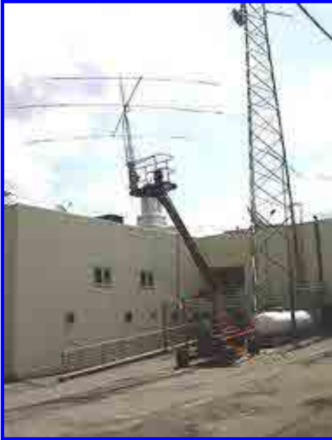
The A3S, 40m sloper off the tower, and a 2m antenna on a pole in the corner of the fence.
