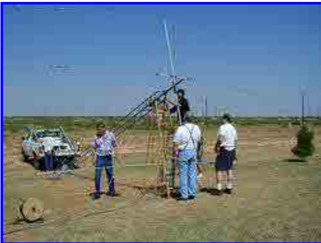
KK5ZG, KD5VOW, KB5RTL, N5ATO, N5RZ, & K5KUX installing the CW station antenna.
