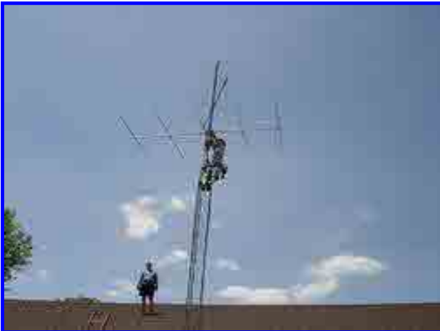
Bill KC2CNB putting the final touches on the VHF tower and antennae, the 6m loop at top is used when the band is hoppint as move the beam takes too much time !
