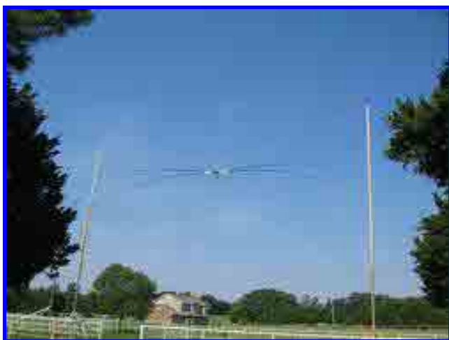
A Moxon rectangle suspended at 40 feet with interchangeable elements for 40, 20, 15, and 10 meters.
