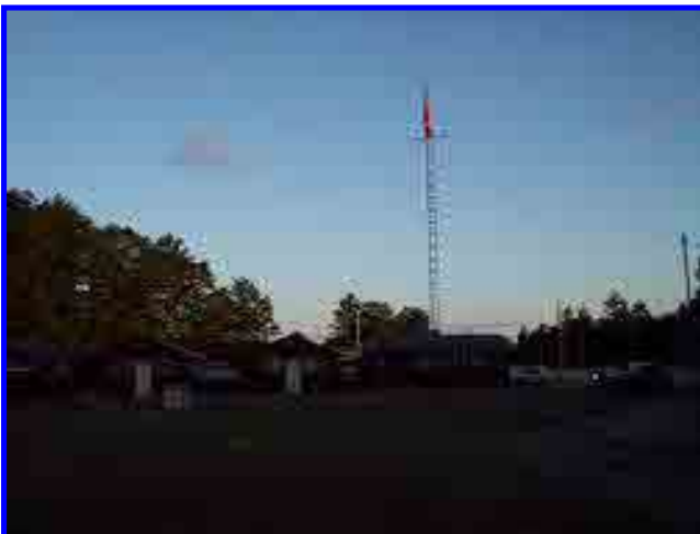
Field Day site at sunrise with 40' tower supporting 40 meter loop, G5RV, and 2 meter beam
