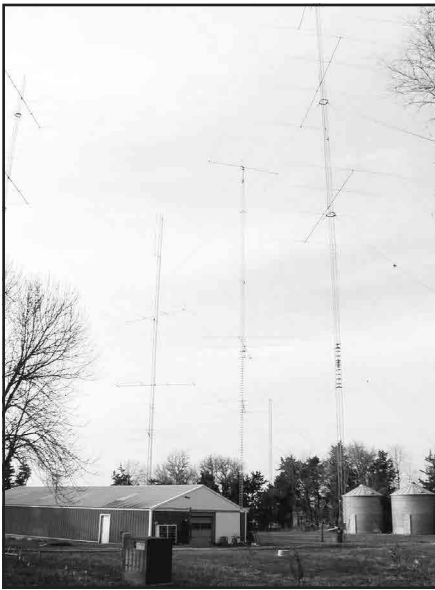
A view of the NØNI stacks
