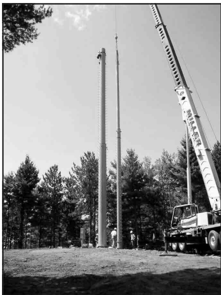
Figure 1—Big Bertha halfway up, installation by Custom Metal Works.
