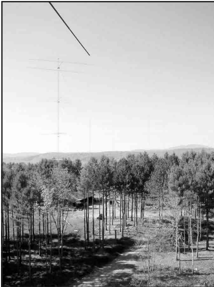
Figure 4—Vermont fall colors frame 160 meter four-square and rotating tower with Force 12 80 meter Yagi and stacked M 2 LPDAs.
