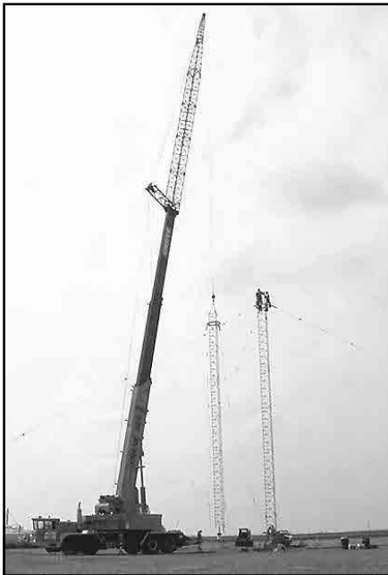
Putting the second 60 foot section up.
