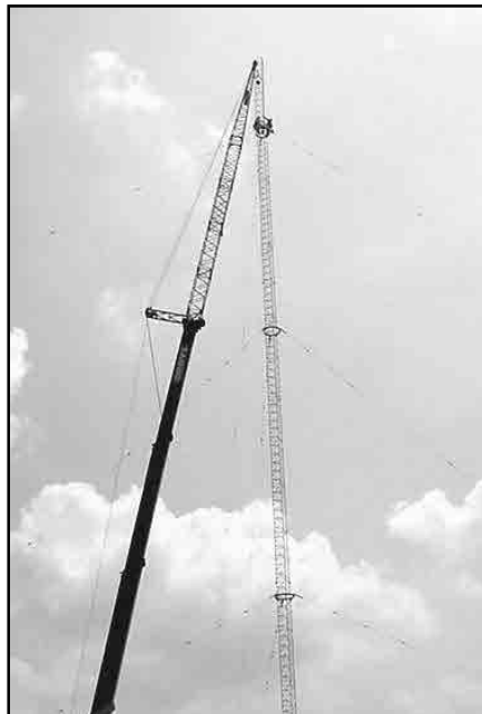
Finishing the new tower.
