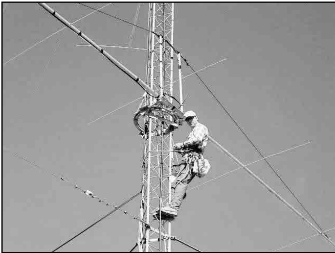
Figure 3—Rick N5DXT completing the installation of the lower 6 meter 2WLC at 36'.
