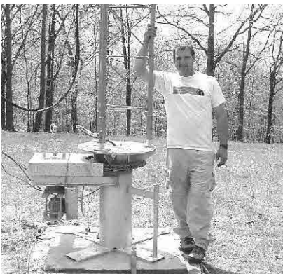
Ground mounted base for 300 feet of Rohn 55G/AB105.
