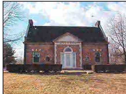
The historic W1AW building, which dates to 1938.
