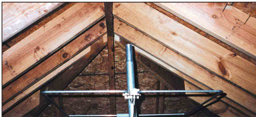
Figure 1—The 6 meter loop mounted near the top of the roof.
