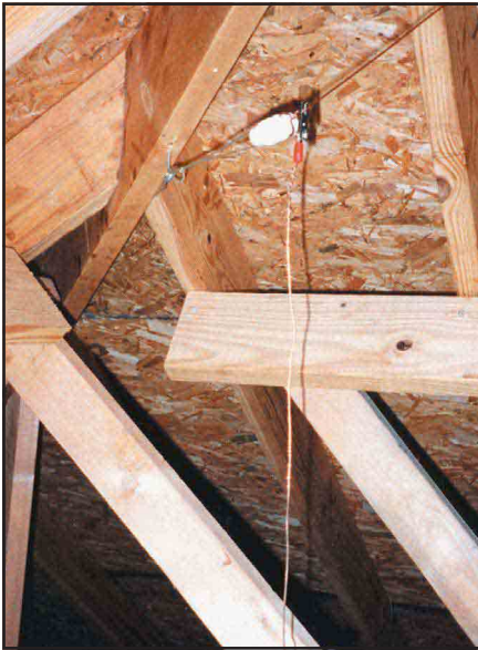
Figure 5—The 10 meter dipole is lengthened for other bands with a simple extension on both ends. An alligator clip secures the extended element.
