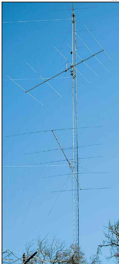
A single tower (this one's at N6RO) can support quite a number of antennas, but care and caution need to be taken when raising the support structure and antennas.
