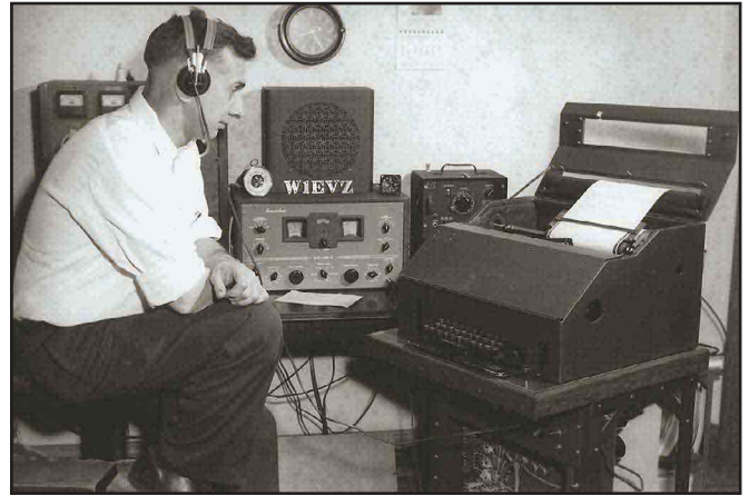
Jim King, W1EVZ, from Holyoke, Massachusetts sent this photo to confirm a QSO on August 27, 1952 with W2JAV. Jim was using a Model 12 Teletype and a Hammarlund HQ-129X receiver. Behind him is his homebrew transmitter. This contact was on VHF, as HF RTTY was not permitted at that time.
