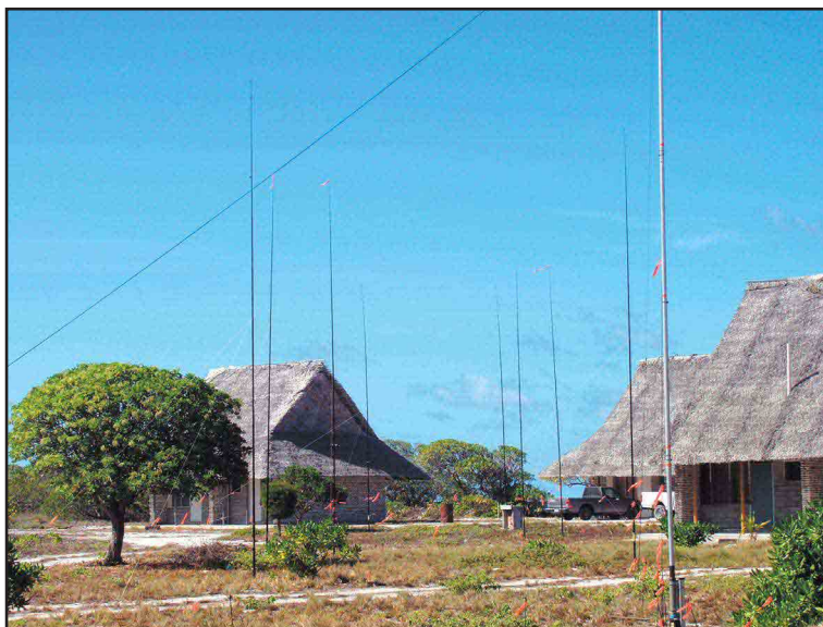
Figure 3—The PVDAs, with the 160 meter vertical in the foreground.
