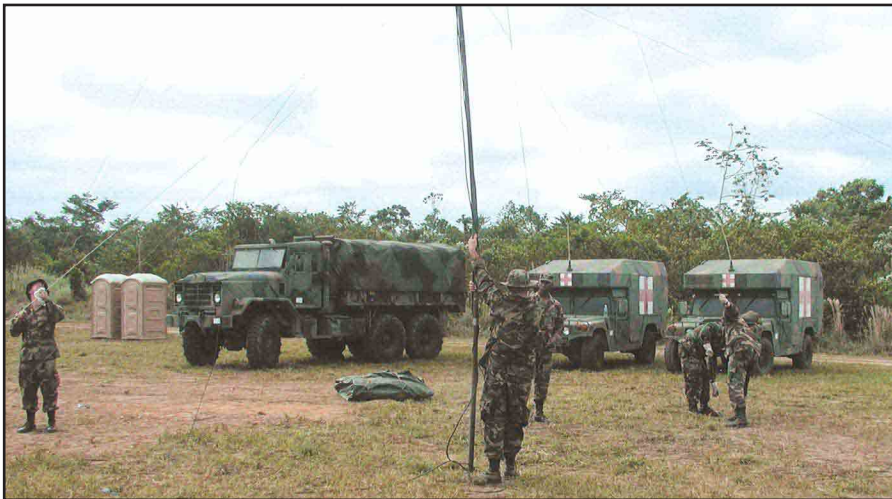
Soldiers erecting the antenna mast that supported the tactical SINGARS antenna and the inverted-V dipole for the MARS station.
