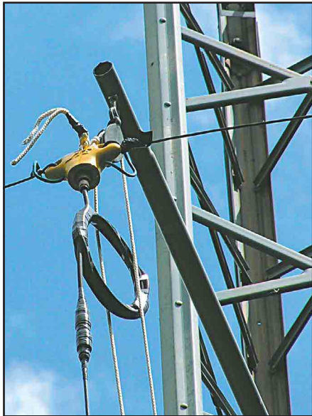
Figure 2—The center of the modified antenna is shown hanging from a tower cross arm. Note the matching length of transmission line (described in the text) wound into a coil to produce a coaxial choke.
