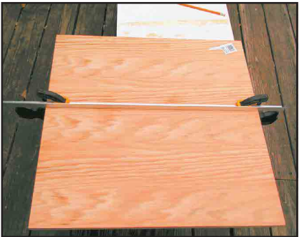
Figure 12—Using a saw guide to ensure accurate cutting.
