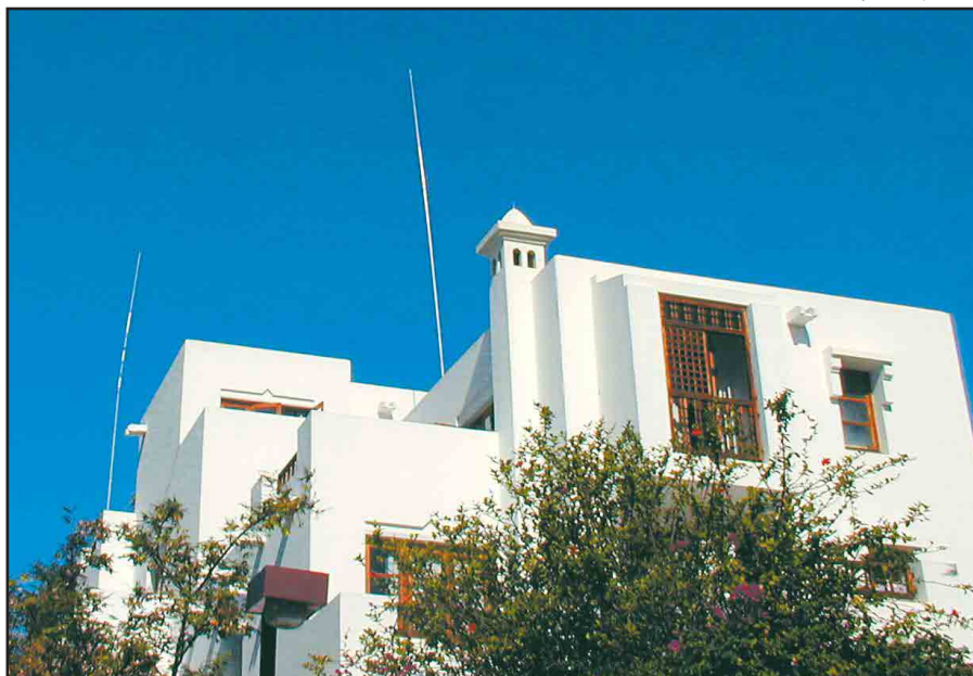
The CN2JS antenna farm perched high atop the resort overlooking the Atlantic just a few hundred meters away.
