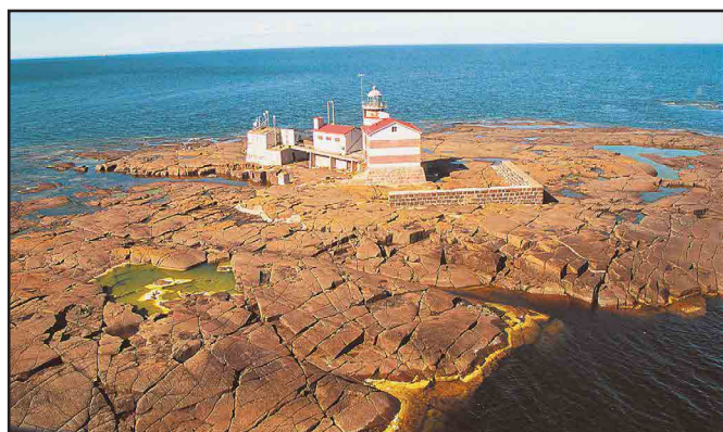
The entire reef of 300 x 80 meters (1000 x 300 feet) has a low profile, and in stormy weather only the lighthouse structure remains above water. Although the light is run by gas, much of the weather-related equipment is powered by solar panels. The reef is divided between Finland and Sweden.
