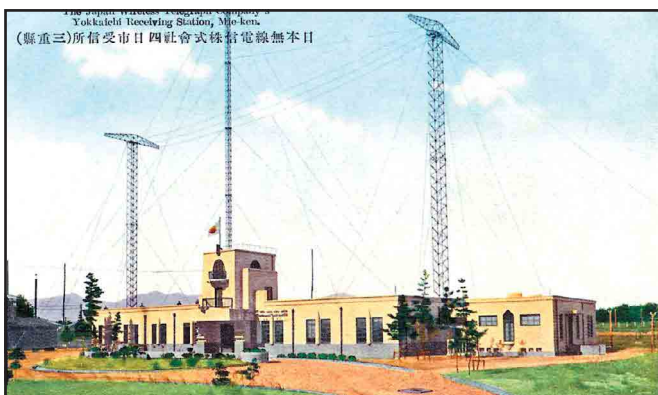
Figure 6—Yokkaichi Receiving Station, Mie-ken.
