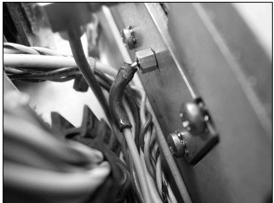
Fig 2—Detail of added feedthrough insulator.
