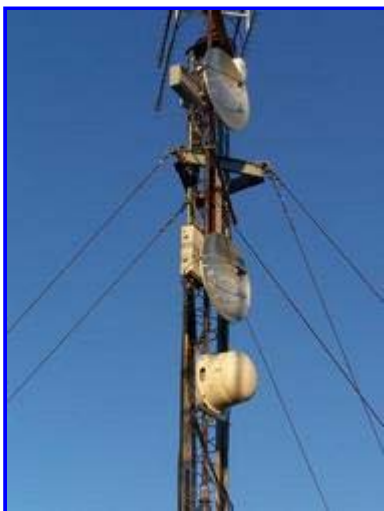
The 10 GHz dish is mounted on the top of a sidearm, with 5 GHz below it, and 24 GHz on the bottom. The box behind the 10 GHz dish houses the transverter and 20 watt power amplifier. IF feedline is a run of 3/8" heliax. The rig downstairs is an Elecraft K2 which makes a nice compact and great CW Rig.
