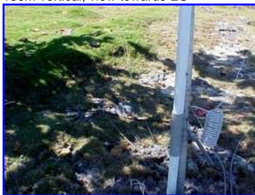
Base loading coil & "gin pole" used to help raise the vertical
