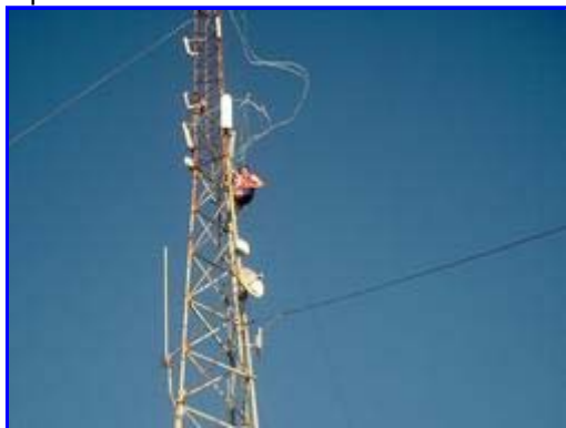
David (K3LP) installing the wire antennas on the commercial 100' tower at the FS5UQ hill top station in St. Martin
